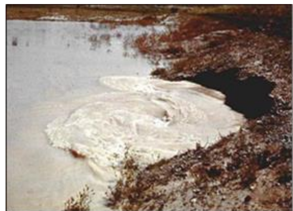
Figure 4-16. Photograph of a whirlpool along the upstream slope of an embankment dam.
