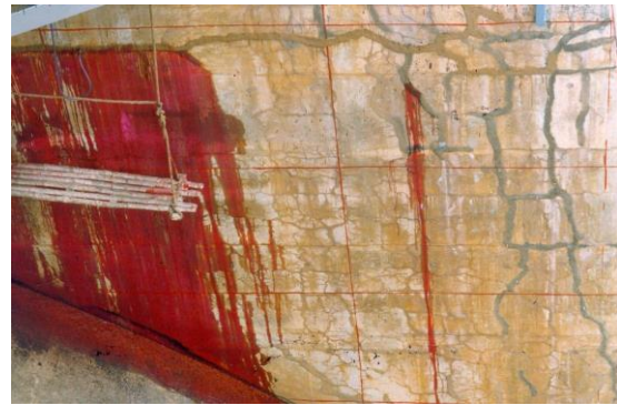
Figure 5-4: Positive identification of ASR at Rihand Dam, India using red dye to demarcate areas of cracks and seepage. no known cure except to minimise exposure to moisture to slow down reaction.
