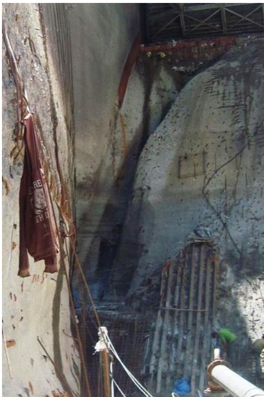
Figure 5-5. Abrasion and cavitation of Gate 1 of Maneri Dam, Uttarakhand, after severe 2013 flooding. Reservoir silted up to the spillway crest elevation allowing boulder-size and quartzite material to flow over spillway.
