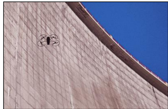
Figure 8-4. An inspection drone at work photographing the downstream face of the Tseuier Dam in Valasi, Switzerland
