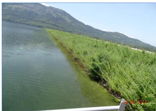
Figure 4-12. Woody vegetation on the embankment is detrimental to the health of the dam by creating seepage paths along the roots and overall impedes dam safety inspections.
