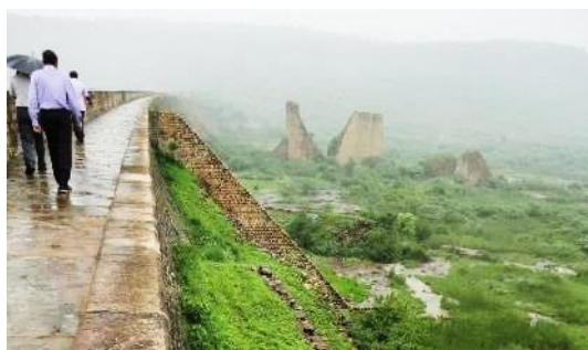
Figure 5-7. During construction (which began in 1916) the dam had a breach in 1917. Causes of the breach noted uplift pressures on a thin clay lens in the sandstone. As a result, methodically placed buttresses were constructed at various chainages along the length of the masonry. (Tigra Dam, MP)
