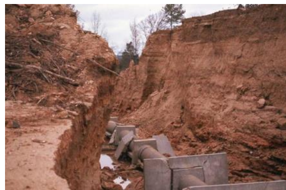
Figure 6-4. Failure of embankment dam resulting from piping erosion along conduit. Compaction around seepage collars is difficult and creates an easy path for water to flow that will initiate backward erosion and carrying of fines. Approximately 25 percent of all embankment dam failures are a result of internal erosion or backward erosion (piping) associated with conduits.
